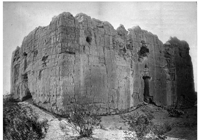
Figure 3: Large scale puddled adobe architecture: West wall of the Casa Grande ca. 1880 | Photographer unknown
